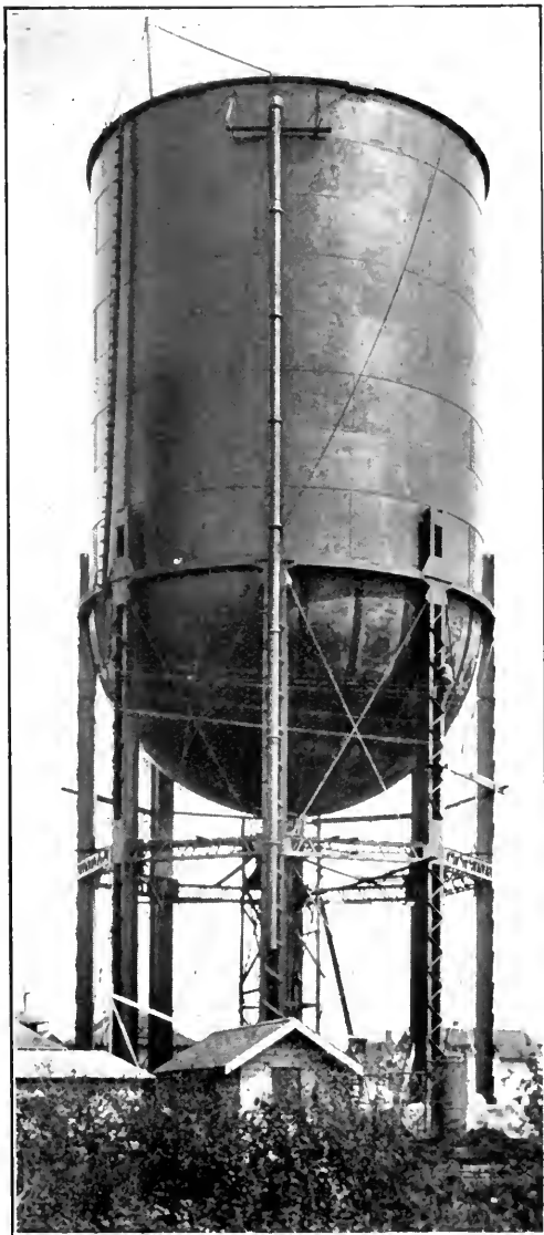
A 1,000,000-GALLON ELEVATED WATER-TANK IN PORTLAND, ORE.
